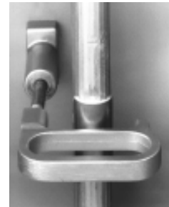
Rung protector installed showing proper placement.
