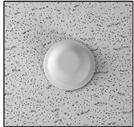
Concealed Sprinkler and Adapter Assembly (Protective Cap Removed)
