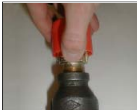
Figure 3: Sprinkler cap being removed from an upright sprinkler.
