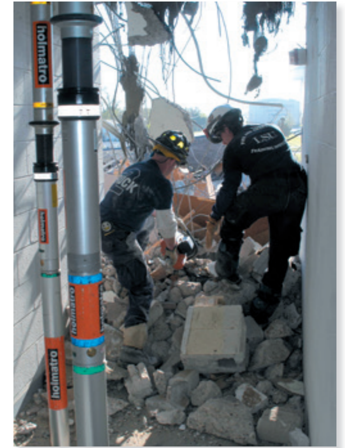
Collapsed building stabilization with a manual Locknut system.
