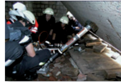
Collapsed structure stabilization and lifting with a hydraulic Locknut system.
