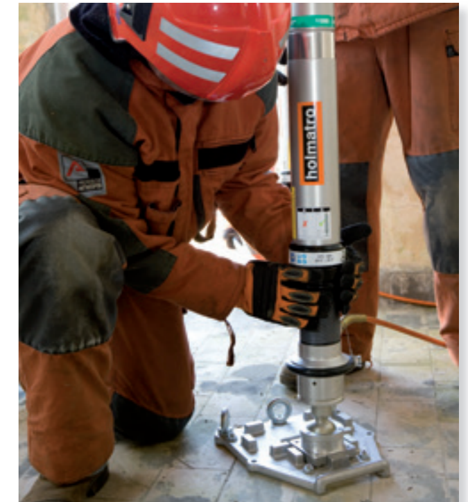
Pneumatic Locknut strut used as a manual strut to shore a building.
