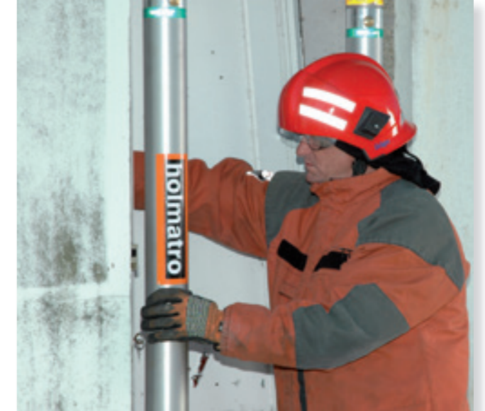
No protruding parts.
