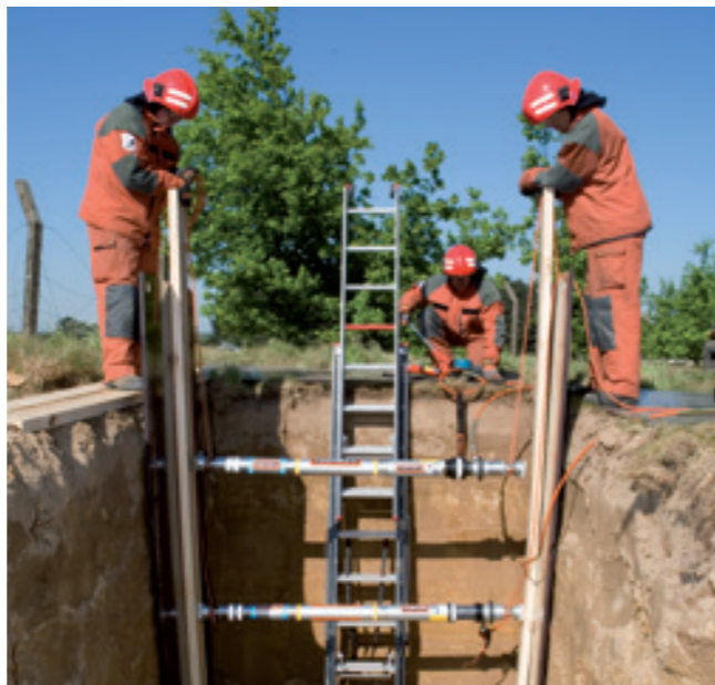
Remote shoring with hydraulic Auto-lock struts.
