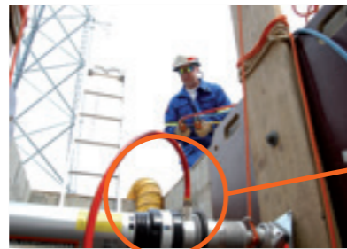
The Auto-lock system enables remote shoring.
