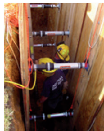
Trench shoring with pneumatic Auto-lock struts.
