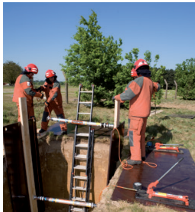
Hydraulic Auto-lock struts used for remote shoring.
