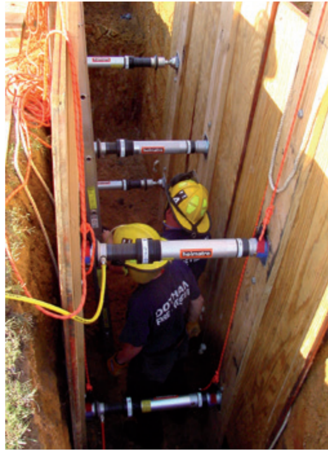
Trench shoring with pneumatic Auto-lock struts.
