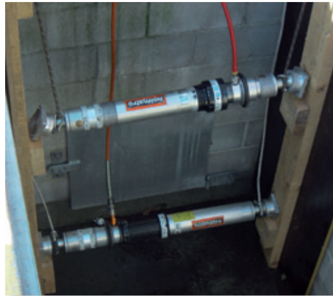
Remote shoring with Auto-lock struts.
