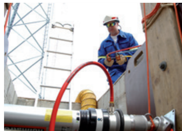
Remote shoring of a trench.
