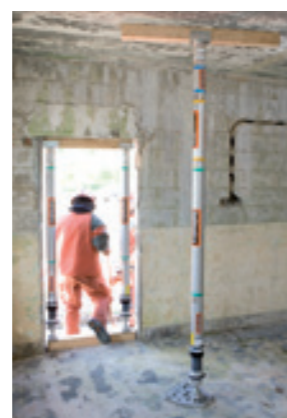
Spot shore used to protect an exit route.
