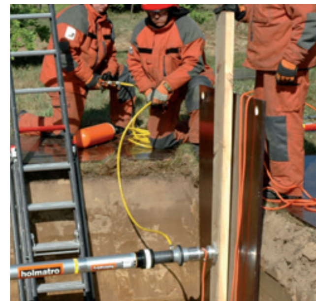
Pneumatic Auto-lock struts are very suitable for remote shoring in trench rescue.
