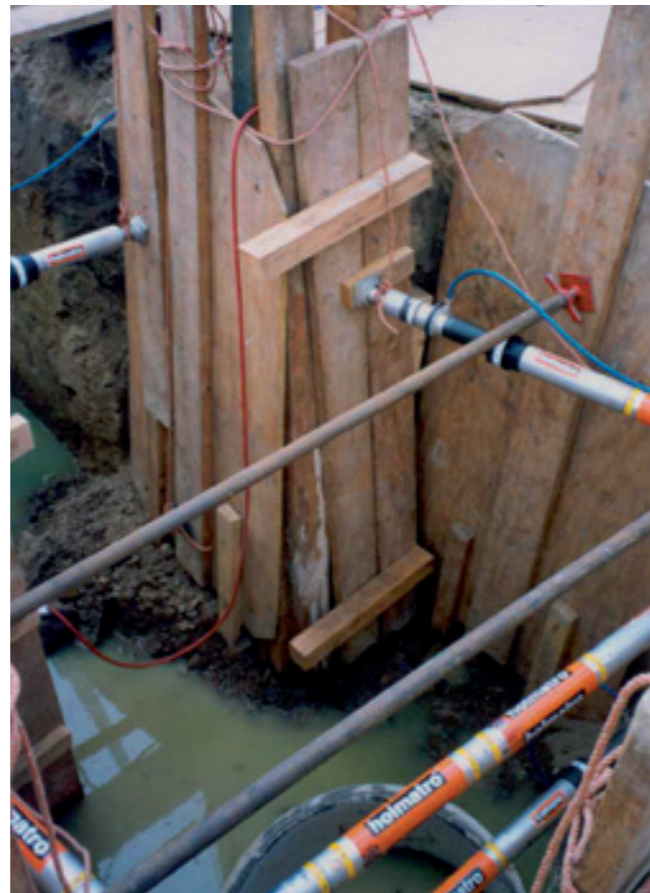
Pneumatic Auto-lock struts positioned in a trench.
